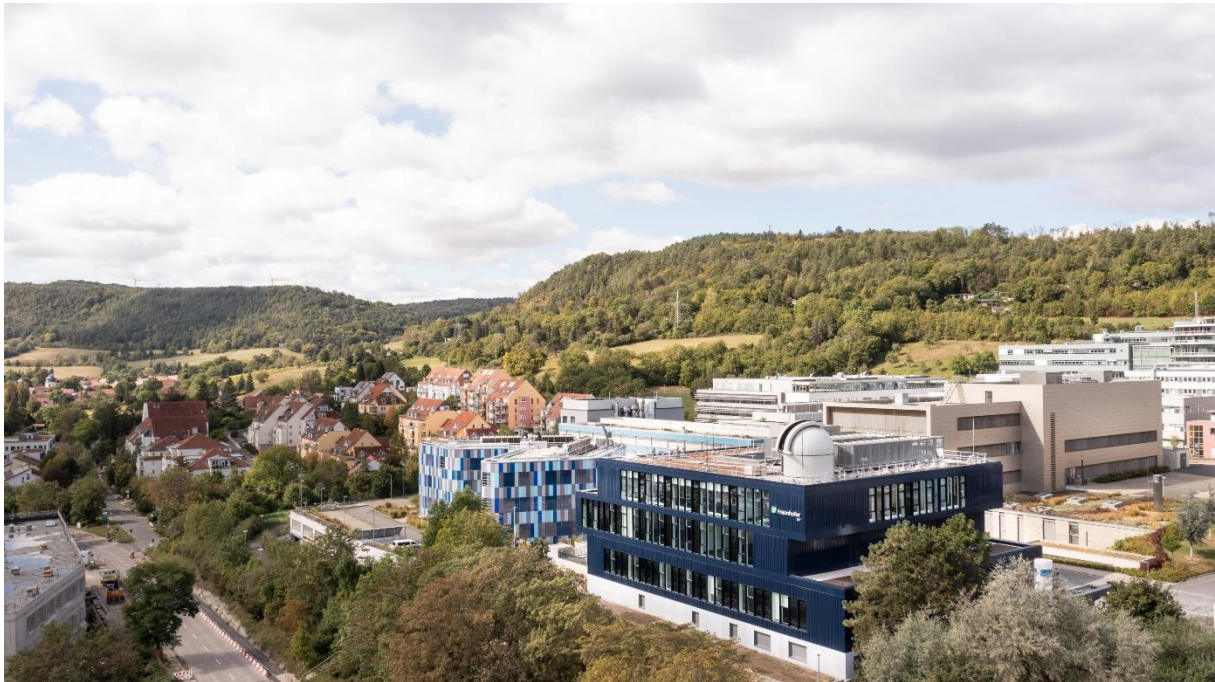
OGS on Fraunhofer IOF Rooftop
